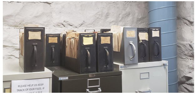
North wall with HVAC duct
