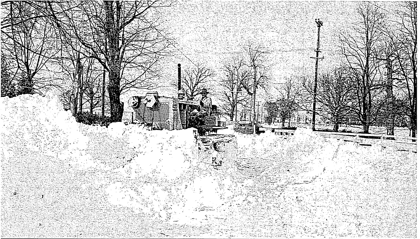
In an earlier era, snow was left where it fell, often making roads impassable until winter had passed and the roads dried out. Anticipating a major snowfall was a bit less predictable in the era before sophisticated weather forecasting. Keeping roads free of snow became a responsibility of the state's highway department after the state government reorganization of 1936. Large sized road scrapers or bulldozers were the preferred means of getting the job done in the early 1950s, as this central Kentucky view suggests. (This photograph is from the Department of Public Information collection of the State Archives holdings, in the Public Records Division, KDLA.)
