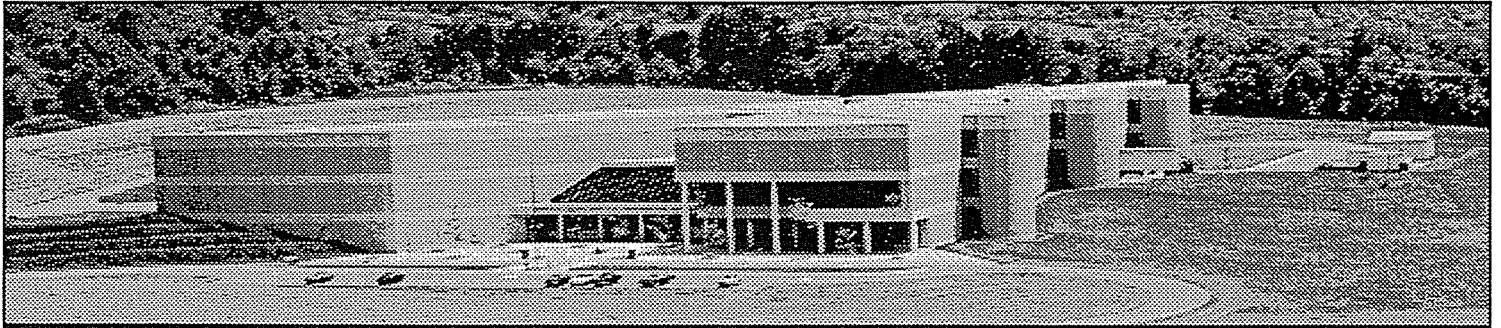
Libraries and Archives' hillside location offers ample room for expansion, evolution as KDLA strives to keep pace with new demands for information and records services made possible by electronic technology.
